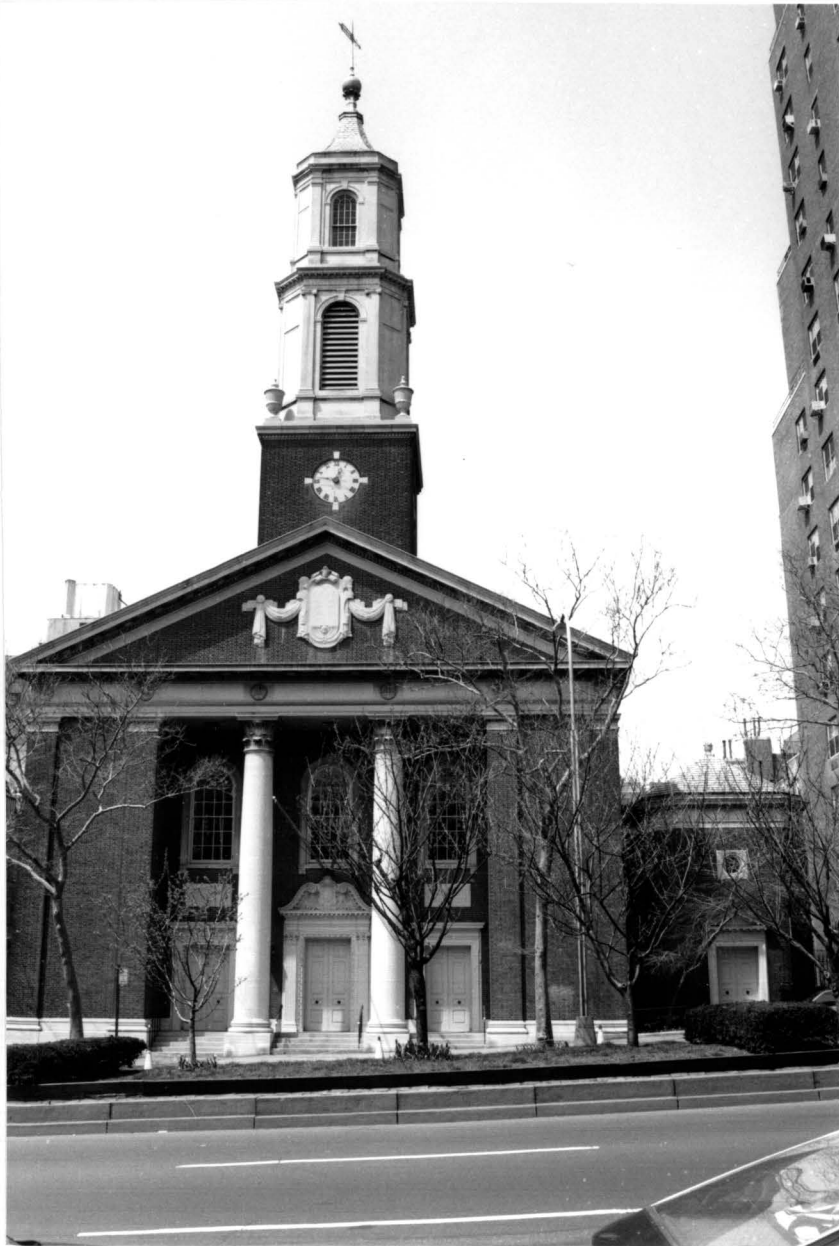
Fig. 44. Brick Presbyterian Church, 1140-1144 Park Avenue (1938-40).
