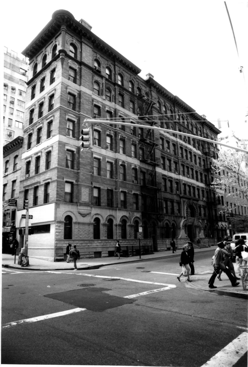
Fig. 14. Hotel Graham, No. 22 East 89th Street (1891-93).
