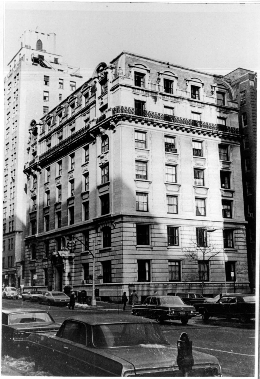
Fig. 36. No. 1261 Madison Avenue Apartment Building (1900-01).
