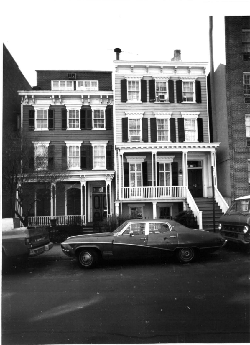
Fig. 4. Nos. 122 and 120 East 92nd Street (1859, 1871).
